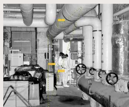
Point cloud data of a mechanical room. While it resembles a photograph, each point in this image is a three-dimensional (3D) coordinate. With the SCENE software, the user can obtain the exact dimensions of relevant parts.
