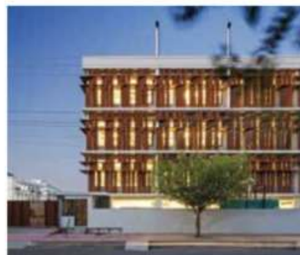
At the Visage Corporate Office in Noida, ceiling fins paired with carpeting lifted sound comfort throughout the floor plates
